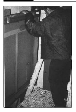
■ Push the Door Panel against the guide bolts. If both side angles on the Door Panel are flat against all the guide bolts, twist is not present. You may proceed with installation.
